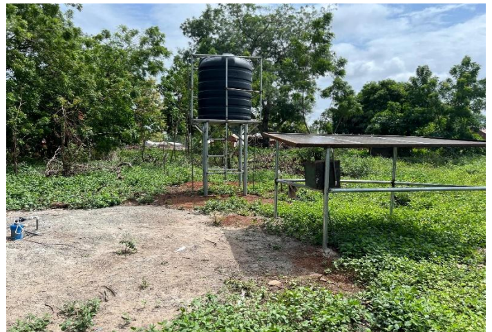
Figure 9: Solar mechanized borehole 2
