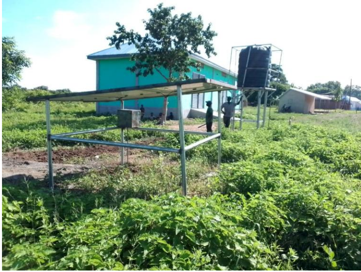
Figure 4: Solar mechanised water system for Nsuidom cooperative union shea processing unit at Manyini community.
